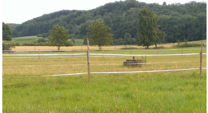
Figure 3-26. Typical facility for drinking water extraction from springs; in maps one often finds “Wbh.” (Wasserbehälter) as its topographical signature.
