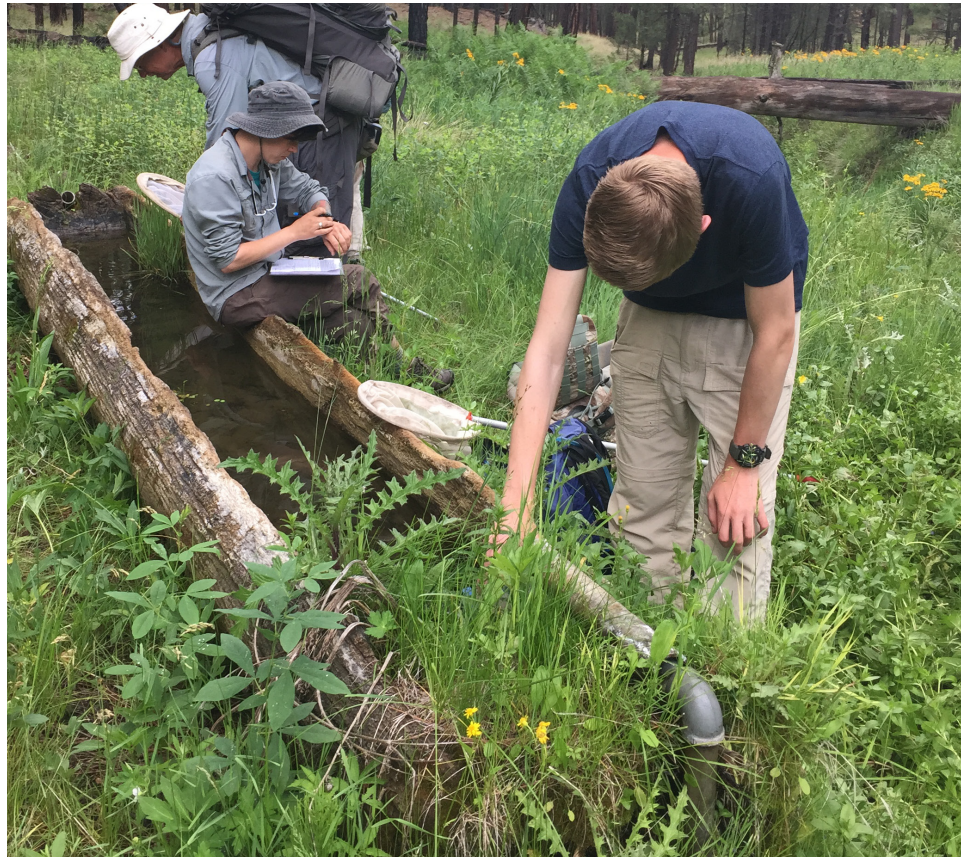
Fig. 1.15: An example of flow splitting at Horse Spring, Apache-Sitgreaves National Forest. A pipeline draws water from the source to a hand-carved wooden trough. Flow splitting draws animals to the trough for water, protecting the source of the spring. Photo by Molly Joyce © 2015.
