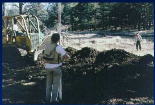
Earth moving, November 1998
