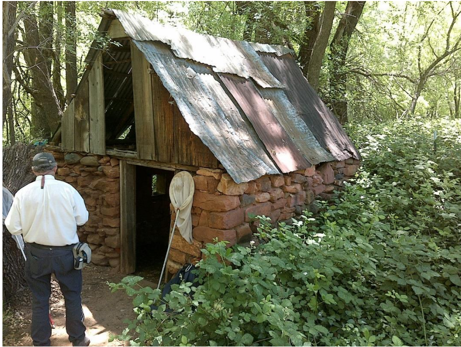
Fig 30.2 Thompson Springhouse Spring: The historic springhouse, as viewed facing south
